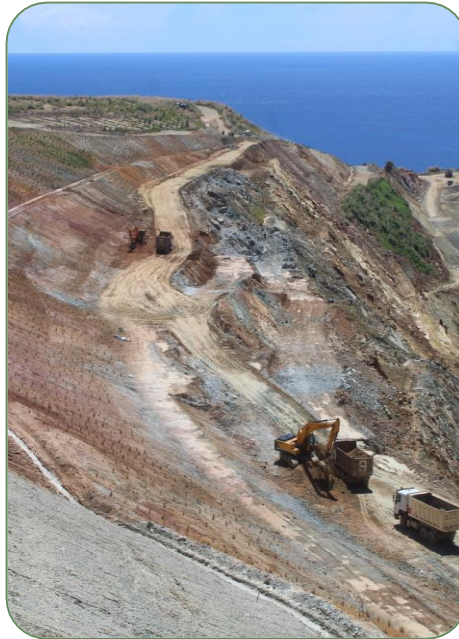
Reconfiguration of North wall Open pit to flatter slope
