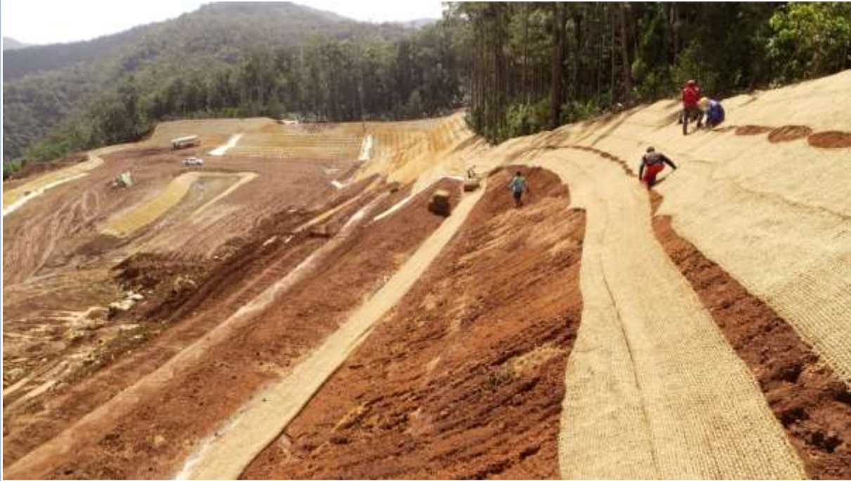
Installation of Coconet
