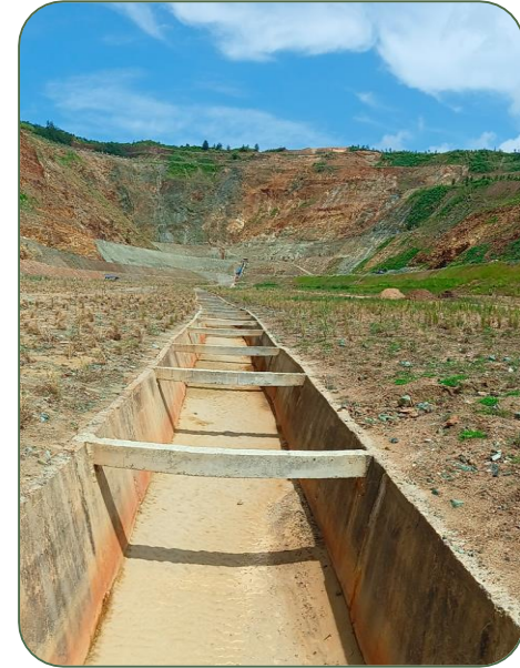
Concrete canal constructed in all areas with prominent flow of water
