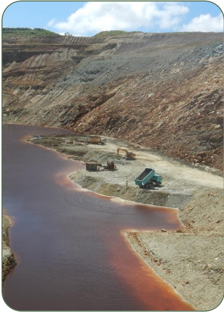
Backfilling of Open pit up to 95mRL
