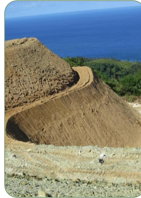
Re-sloping/grading the embankment of TSF
