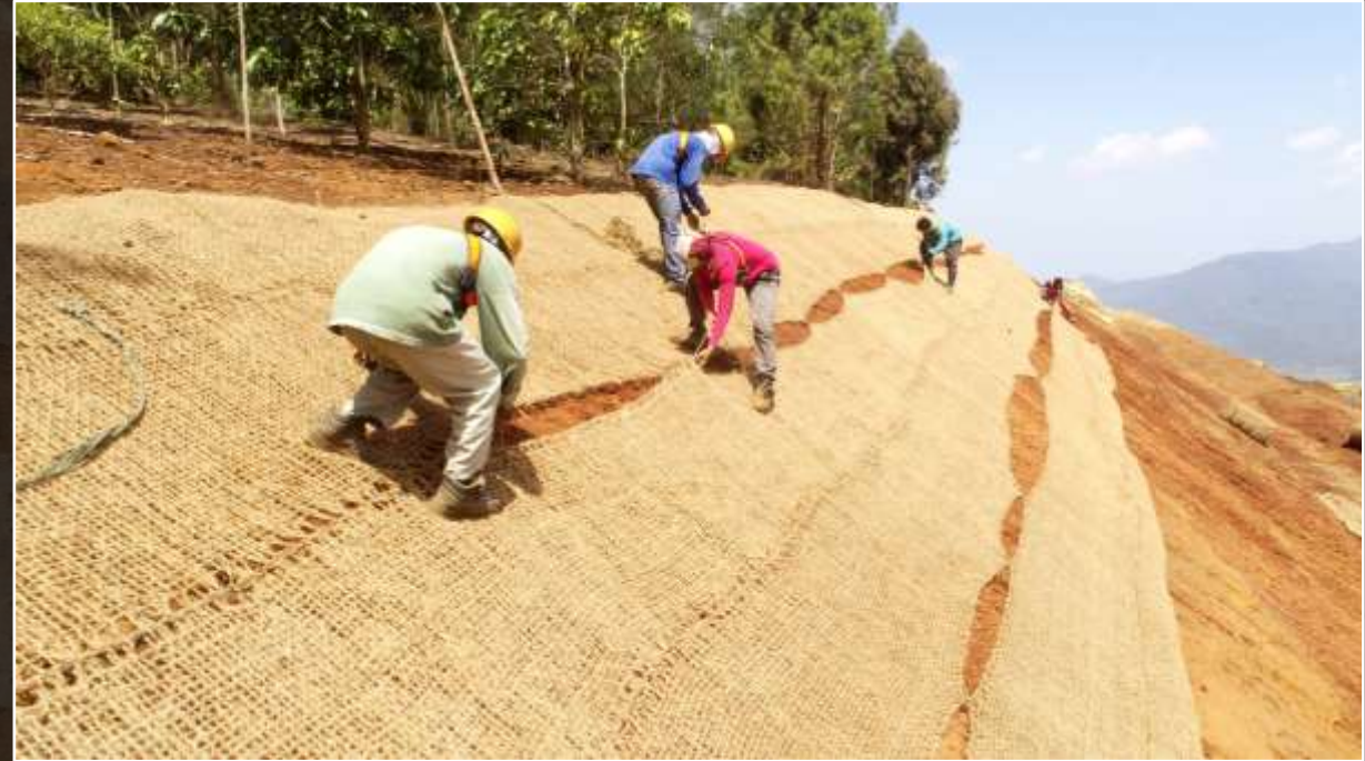
Installation of Coconet
