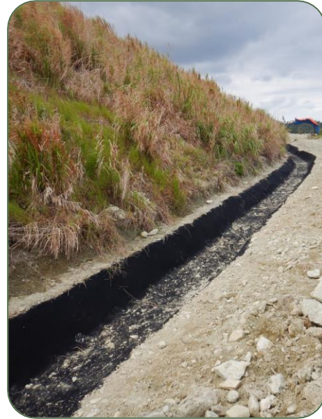
Geotextile matted ditch prominent at TSF embankment
